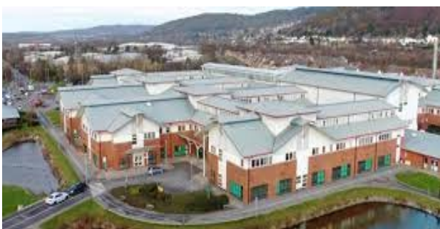
Neath Port Talbot Hospital, Port Talbot
