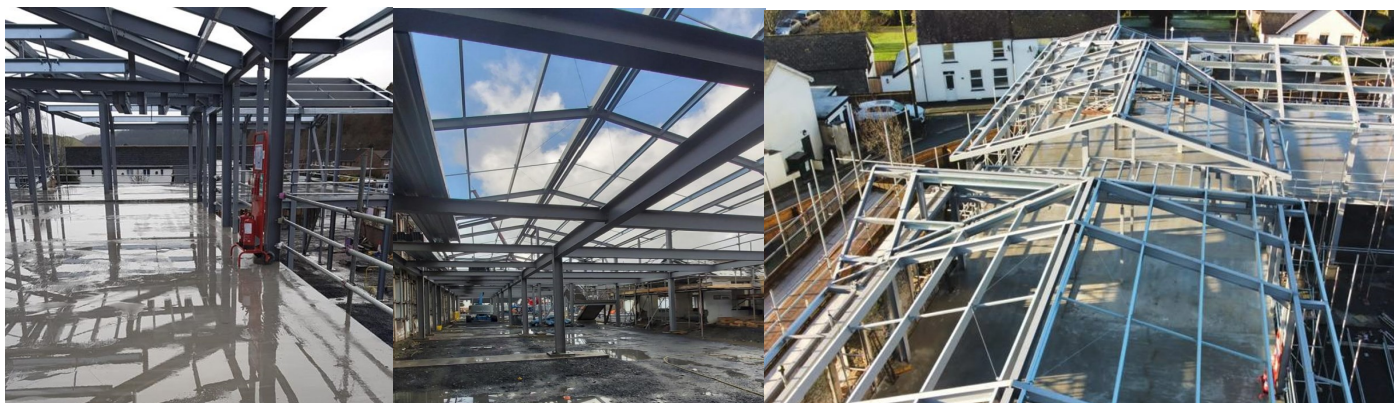
January Progress Photos - Steel Frame Erection
