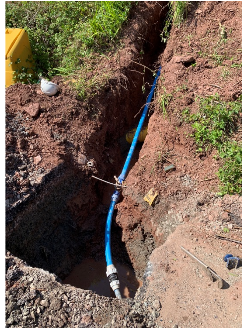
Replacement of failing water supply mains and distribution pipework at Bronllys: £31K
