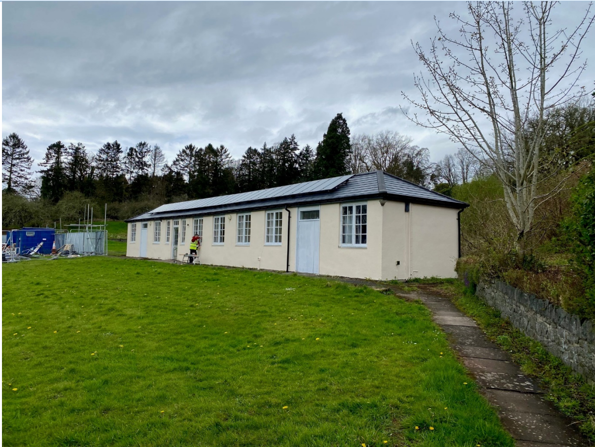
Following outside refurbishment.
