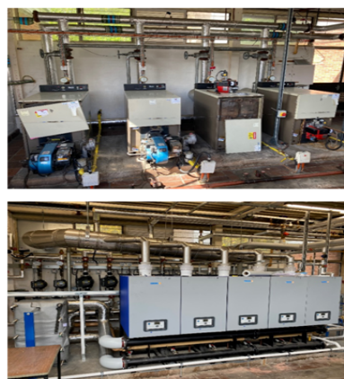
Replacement boilers: Newtown (before & after)
