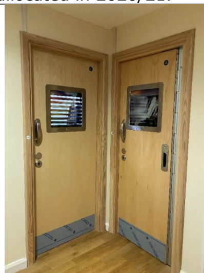
Progress photos: Bryntirion upgrade and anti-ligature doors at Felindre Unit, Bronllys
