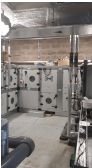
Replacement Endoscopy air handling unit in roof top plant room with appropriate access stair
