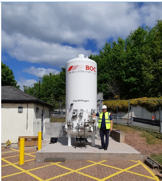
Oxygen VIE installed Brecon
